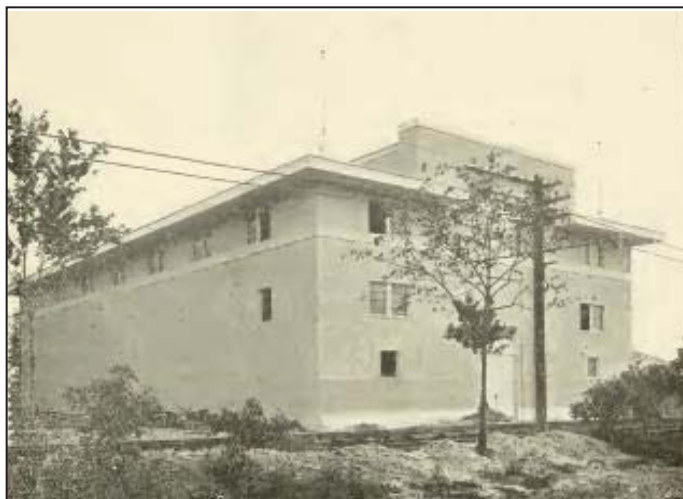
The Aeronautics Building at the Jamestown Exposition of 1907 was the first building in the United States dedicated to the construction, display, and preservation of aeronautical objects. Photo from the American Magazine of Aeronautics, July 1907.
